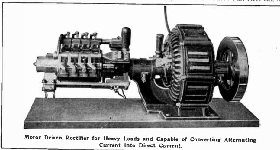
Motor Driven Rectifier for Heavy Loads and Capable of Converting Alternating Current Into Direct Current.
