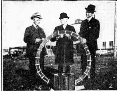
Fig. 1. Lowering Secondary Coil Into Place on 10,000,000 Volt Transformer. Fig. 2. Mr. Thordarson, Designer of Mammoth Transformer and One of the Secondary Sections.
