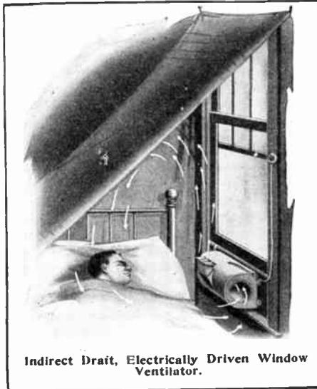
Indirect Draft, Electrically Driven Window Ventilator.
