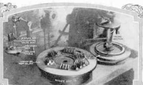
Machinery for finishing automobile parts with a nicety as great as those finished by hand is il-lustrated on this page. Left: One rotary section of the machine is used for refinishing flat unrestricted surfaces and for truing lapping sticks.
