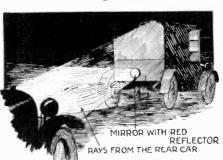
In case your tail light should go out, you need not be afraid of a rear-end collision if your car is equipped with a red-backed mirror as shown above. Approaching headlights will be reflected toward the driver of the coming car, thereby warning him.
