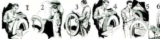
Successive stages in retreading tires: 1—Old tire painted with a special liquid and 2, heated with torch flame. 3—Charred rubber is scraped off, rubber being devulcanized. 4—Vulcanizing liquid applied, and at 5, new rubber is put on tire. Tire is put in mold, 6, and cured at 7.
