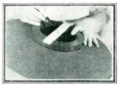
The hole in the cross bar through which the connecting rod passes should be accurately centered to avoid friction.
