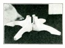
When both base members have been cut out and smoothed, it will be found that they fit together as shown above. It may be necessary to retrim the edges to obtain an accurate fit.
