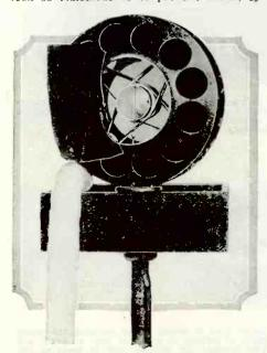
Here we find a photograph of the microphone which detects sour notes. The aluminum cup is supported on the inside of a studio microphone case. The snake fits into the cup.
