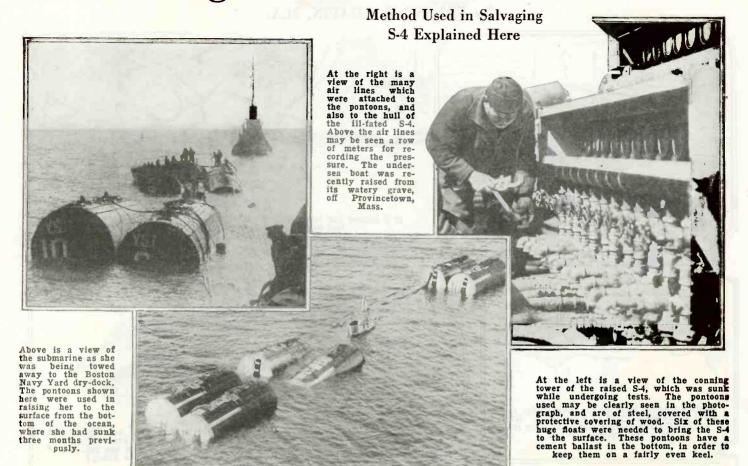
The submarine S-4 was raised in much the same manner as was the S-51 some time ago. In both cases, pontoons were used and the submarine hull was blown out with
