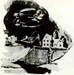
The above illustration shows a new style of proposed heli-copter which has a separate engine in each of the vertically acting foils and also an engine and propeller for propulsion.
