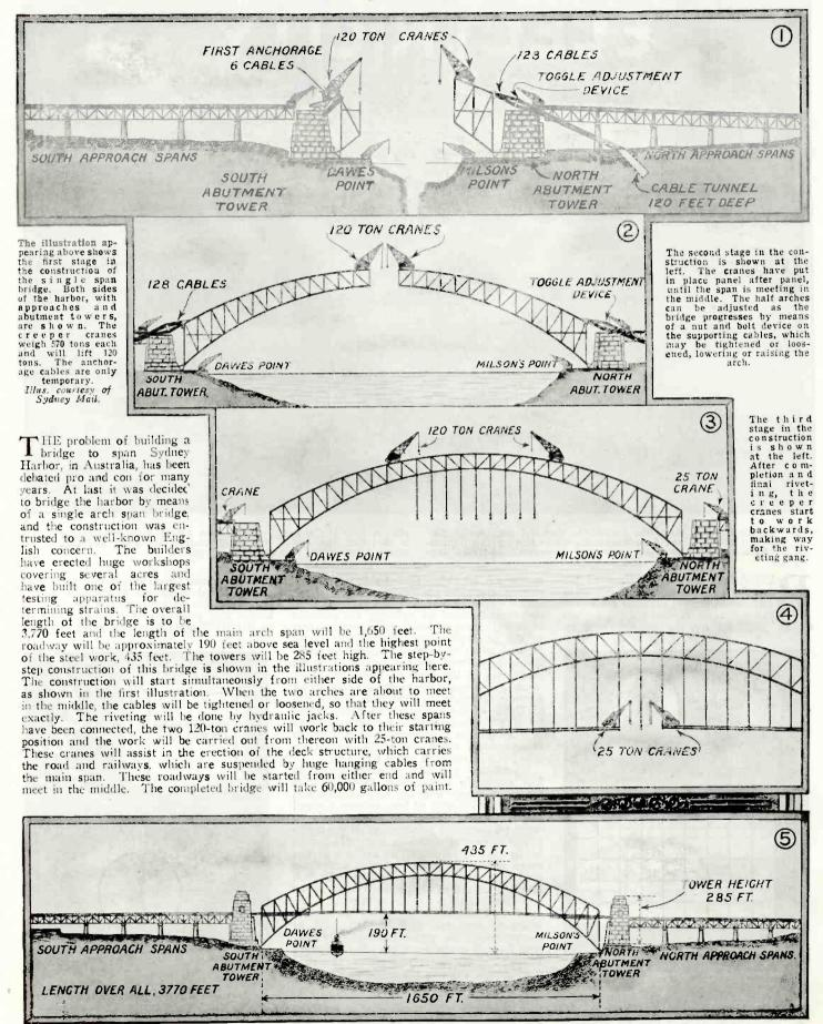
The fourth stage in the construction is shown and consists in building the road and railways. The completed bridge is shown directly above.
