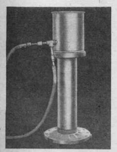
The above photograph shows the furnace ready for work. The stand is made from a section of 8-inch pipe with a flange at each end.
