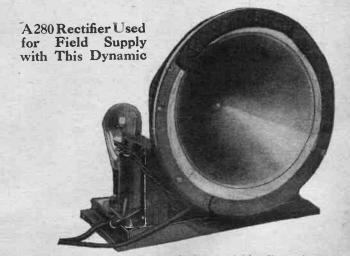
Fig. 3. The speaker shown above obtains the field coil supply from a 280 type rectifier which supplies direct current. The transformer and rectifier tube may be seen at the left.
