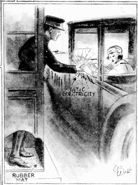
Holland Vehicular Tunnel collectors were recently insulated against static electricity. They had complained of shocks to their hands when collecting the tickets from the motorists. The cars coming down the steep hill to the tunnel collected a static charge. Rubber mats have been provided for the collectors. This condition is only found on the New Jersey side.
