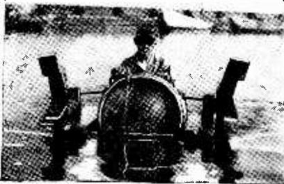
A ten-year-old boy is shown seated in one of these paddle-wheel boats. They are operated by turning the cranks by hand and steered by varying the speed of the two paddle wheels.
