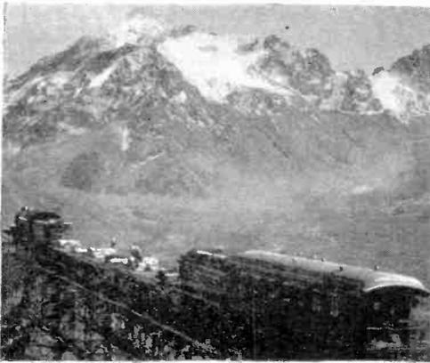
Passing through a land of scenic beauty, mineral wealth, and majestic mountains, the Peruvian Railway crosses the Fiscas Bridge, shown above, located at an elevation of 15,500 ft. Water at this altitude boils at about 134° F., and the number of thermal units is lowered proportionally. It is usually necessary to have special combustion chambers to offset this lowered efficiency.
