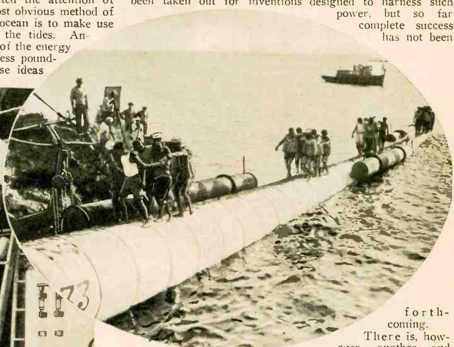
Above — Showing the final successful launching of the mile-long tube from small flat cars running down to the water's edge on a narrow gauge railway. Expert swimmers from the Cuban navy assisted in the launching. Left — The hot water purifier and the boiler in which steam is generated.
