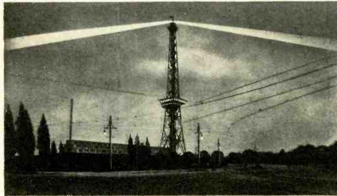
Night view of Witzleben Tower, Berlin. On top is an aviation beacon and observation gallery. One third of the way up is a restaurant. The tower supports the aerial of the Witzleben broadcasting station. Below the tower can be seen the stepped roof of the Radio Exhibition building, which housed the television apparatus.
