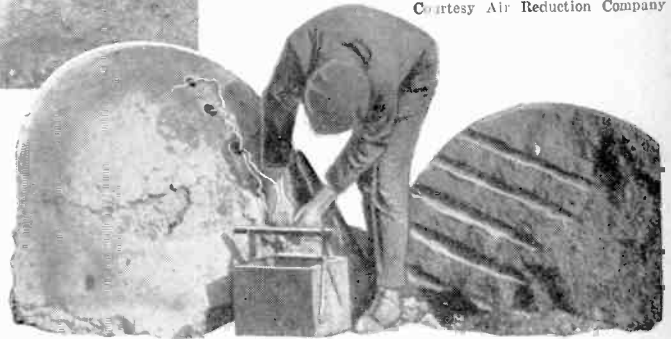
Preparatory to blasting a skull, holes are burned into it with pure oxygen delivered by a \frac{1}{4} inch gas pipe.
