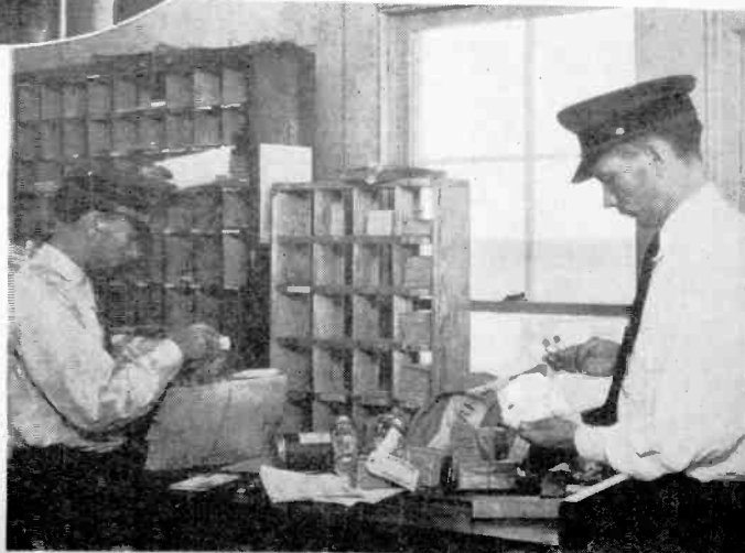
Inflating a pilot balloon preparatory to making upper air investigations. These balloons are used to ascertain wind direction and velocity at the different altitudes.
