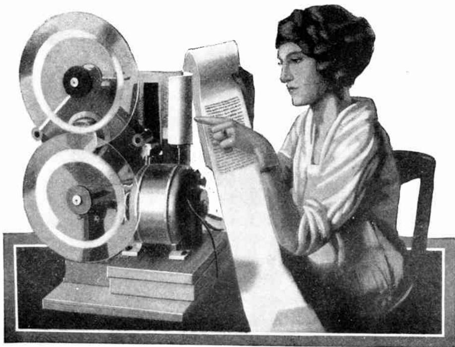
Machine for transmitting typewritten copy on long strips as a continuous process. A hundred words a minute is not difficult, and one thousand words a minute will soon be possible, it is believed.
