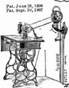
By attaching an adjustable Water Motor and Water Fan to your water pipes, you can make your life more comfortable without expense.
