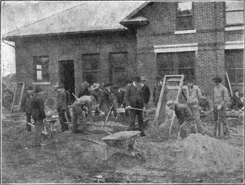
Fig. 1. Method of Screening Sand from Gravel
