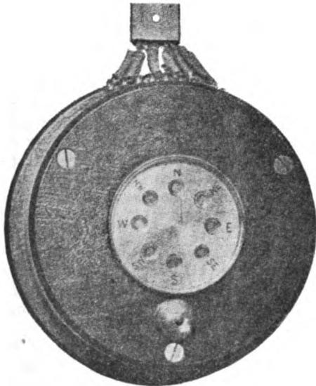
Photograph of Wind Vane Electric Indicator
