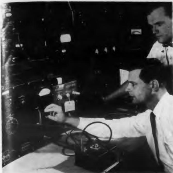
Mounted in the foreground is the experimental transistor which can provide 5 w at 10 mc. The transistor is designed with an intrinsic layer of silicon between the collector and other elements, which makes possible its high frequency performance.
