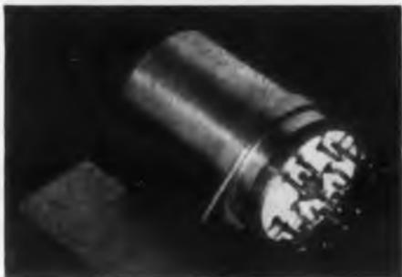
This 4pdt relay has the following characteristics: Operates in an ambient temperature of +200 C, withstands 55 g shock for 11 msec, withstands 25 g vibration up to 2000 cps, and has a contact bounce of less than 250  $\mu$ sec. Insulation consists of all ceramic material in order to maintain high resistance at maximum operating temperature. The coil is hermetically sealed from the contact structure. The relay retains the rotary principle of operation standard in the Company's line of relays.
