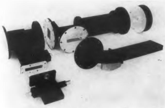
Here is the plumbing associated with the attenuator. At the upper left is the directional coupler and attenuator. To its right are the orthogonal junction, the ferrite rotator, and a 45 degree twist. The dummy load is shown at the lower right and the bolometer mount at the lower left.
