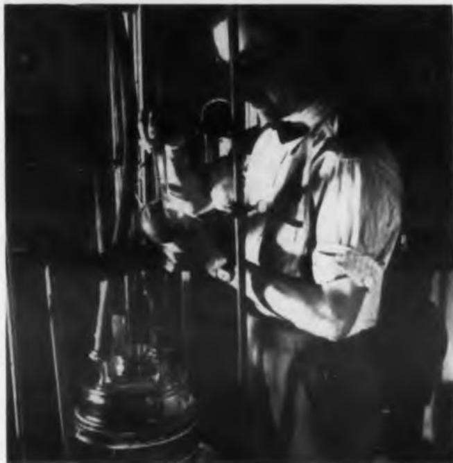
**Atom-by-atom buildup** of the transparent phosphor screens is accomplished with this vapor phase deposition equipment. An evaporation process may be used.
