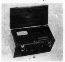
Using thermistor sensing elements, the model 109 temperature indicator covers a range of 60 to 90 C. It indicates temperature at ten different points to 0.1 deg C accuracy.
