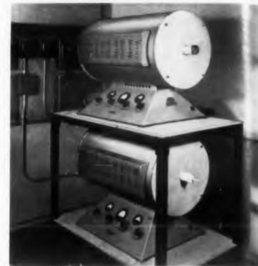
The growth of silicon crystals in an inert atmosphere takes place inside a 2-in. OD quartz tube in the G-02720-PT furnace. The furnace can maintain uniform temperatures up to 2560 F for 150 hours. The crystals are sliced into wafers, then cubes, for use in semiconductors.
