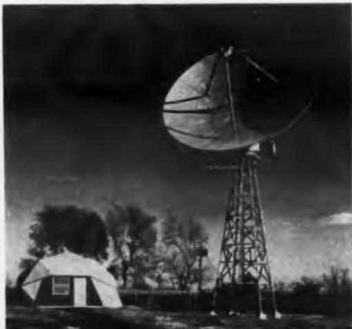
FCC has granted ITT Laboratories, Nutley, N. J., permission to use this 40-ft steerable antenna for narrow-band transmission into space. Moon and passive satellites will be used for studying interference problems as well as checking some performance details of a planned PCM-FM active satellite communications system.
