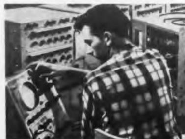
**Time-display systems** for world-wide tracking network indicate elapsed time in seconds, minutes, and hours starting several days before each firing. Displays also show estimated time to subsequent events like orbit, re-entry, etc. Basic standard is extremely stable 1-mc oscillator adjusted to WWV timing signal transmissions. Beckman produced 25 displays for network.
