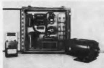
The Reactron is a static ac power-compensating transformer which, in conjunction with silicon rectifiers, provides constant but infinitely adjustable motor speeds, in ratios up to 100:1, on dc shunt-type motors directly from ac power supply. The motor may be operated at full-load torque at all speeds, and up to three times full-load torque intermittently. Units are available with motors in 1/50- through 1-hp models.
