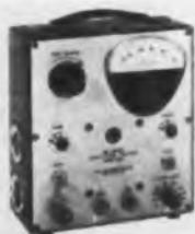
Model HV53 high-voltage-insulation tester has a continuous adjustable output of 0 to 5,000 v rms. It has a calibrated high-voltage circuit breaker with a continuously settable trip-point between 10  $\mu$ a and 3,000  $\mu$ a. It measures 7-1/2 x 3-1/8 x 8-1/2 in. and weighs 8-1/2 lb.
