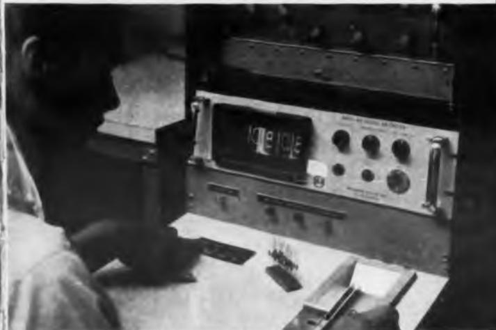
**5** **FULLY AUTOMATIC OPERATION**, pioneered by NLS, includes automatic selection and indication of range and polarity. Human error is virtually eliminated.
