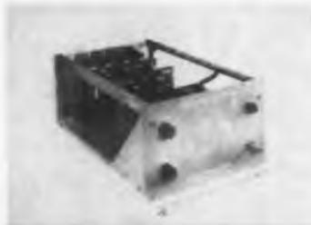
Is transistorized. Model 7 wideband antenna multicoupler operates from 2 to 32 mc, providing outputs for 8 receivers from a single antenna. The solid-state unit has input and output impedance of 75 ohms. Insertion gain is 2 db, noise figure less than 8 db. Input vswr is 1.7:1, output vswr 1.14:1. Unit weighs about 10 lb.
