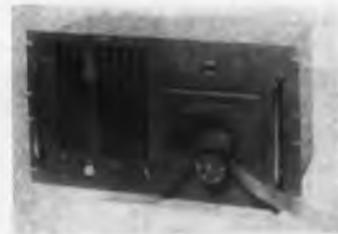
Up to 80 bits of information can be read simultaneously by means of TP 401 tape reader. The unit reads 10 lines and 8 levels across at a time at 6 tests per sec. Special search speed runs at 12 ips. A frame counter indicates the number of frames the tape has advanced from a selected point. TP 401 measures 10-1/2 x 13 x 19 in.
