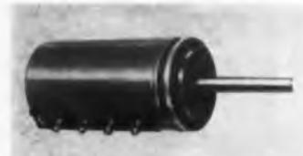
With 10-turn design and a diameter of 7/8 in., series 59M14-10 units have resistance values of 1,000 to 100,000 ohms in linear functions. Standard resistance tolerance is  $\pm 5$  per cent; independent linearity is  $\pm 0.25$  per cent. Power rating is 4.5 w at 40 C. Clarostat Manufacturing Co., Inc., Dept. ED, Dover, N. H.
