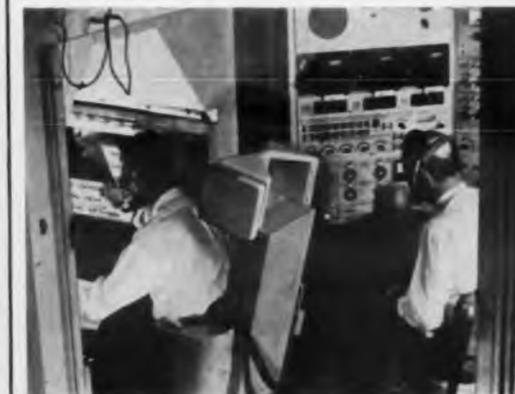
Student and instructor compartments of simulator for operators of B-58 electronic countermeasures station houses equipment for simulating missions, which can be programed automatically. Three punched matrix cards feed program information into trainer from triple box-like device above and to left of instructor, who may change conditions or insert malfunctions.
