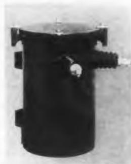
Broad-band balun transformers match 50 to 75-ohm coaxial lines to 600-ohm balanced transmission lines over the hf range. Devices operate from 2 to 30 mc and display essentially flat input impedance vs frequency curves. Model 517 is designed to pass 10 kw cw, and may be pole-mounted. Model 532, a receiving type, passes 500 w.
