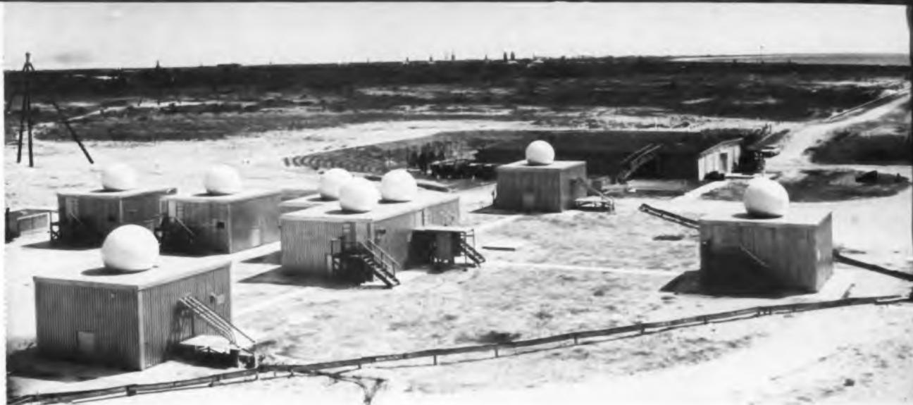
This battery of precision radar antennas—part of the Mark II system—permit the Air Force to track missiles with incredible accuracy. The system tracks a missile by transmitting radio signals to a small airborne transponder which beams a continuous signal back to earth. This signal is captured by these parabolic receiving antennas and sped into a computing system which translates the missile's flight progress on a large plotting board. Azusa Mark II was designed and built by Convair/Astronautics.
