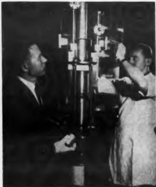
Experimental model of 24-megawatt superpower klystrons, being developed by Sperry Gyroscope Co., Great Neck, N.Y., for a proposed two-mile-long atom smasher, is assembled by Sperry engineers. Energies of up to 10 to 20 billion electron volts are expected to be achieved by driving relatively lightweight electrons along a straight path. Six tubes will be delivered to Stanford University later this year. The accelerator of the atom smasher will require 240 of these klystrons.
