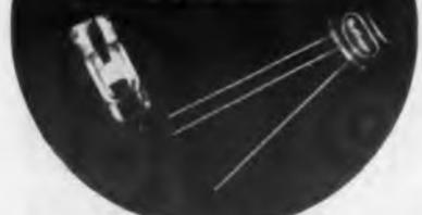
Encased in glass packages, Hoffman Zener Voltage Reference Diodes (types 1N822, 1N823, 1N824) fill the need for highly reliable sub-miniature devices. They are able to withstand severe environmental conditions.
