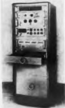
Low-level data signals are displayed and recorded on paper tape by this multichannel digital system, model ER-3295. Consisting of five separate units, the instrument scans consecutively 98 three-wire inputs from various transducers. Resolution is  $\pm 1 \mu\text{v}$ . A digital voltmeter provides visual readout. A slave scanner can be added to increase input capacity.
