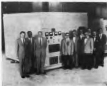
This is one of the 600 KW static, magnetic, rectified direct current power supplies furnished to Brookhaven National Laboratory for use with the 30 BEV Alternating Gradient Synchrotron.
