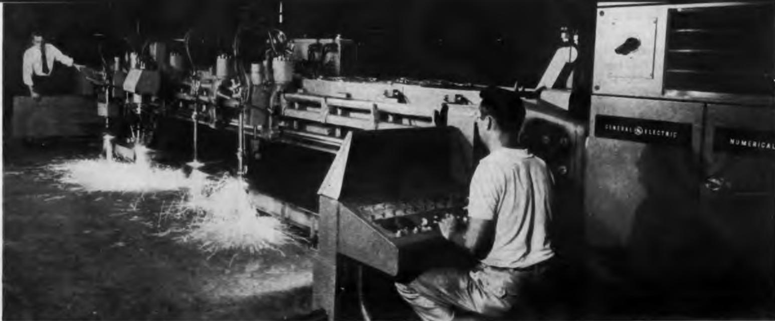
**Automatic control** of four flame-cutting heads is provided by GE's Mark Century Numerical Contouring control for an automated flame cutter built by Air Reduction Co. The solid-state electronic-control system generates slope and circular arc motions from a simplified programming input of desired end point and angular velocity.
