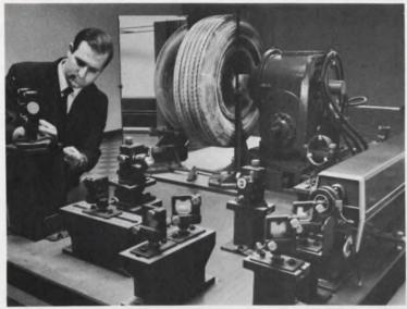
Holographic interferometry, powerful new nondestructive test technique, pinpoints hidden defects in automobile tires. Details on page 25
