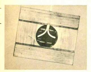
Rear view of the assembled switch showing the bottom strips which holds the wire in place.
