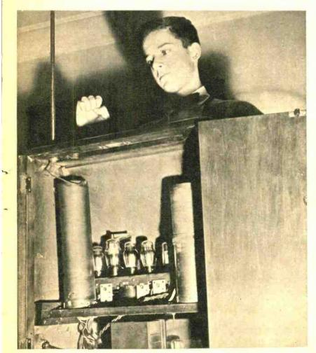
Six tubes, plus power supply (not shown), comprise the original RCA model. Note the variable pitch oscillator coil and pitch antenna (vertical), at left side of cabinet.
