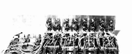
This photograph was taken during construction of our prototype unit. The four input pre-amps may be seen on the right. Directly in front of the pre-amps are the slide potentiometers used for individual volume controls.
