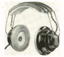
incorporated in each earphone. Since the "Stereophones" have an impedance of 4 ohms they can be connected directly across the amplifier's output or speaker's voice coil and thus no extra wiring within the amplifier is required.
