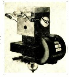
of microwave-oven technology as c.w. magnetrons and power supplies for microwave heating, microwave cavities, mode stirrers, and door-seal designs. Later, patents by *Tappan*, *General Electric*, and *Litton* further advanced the art.
