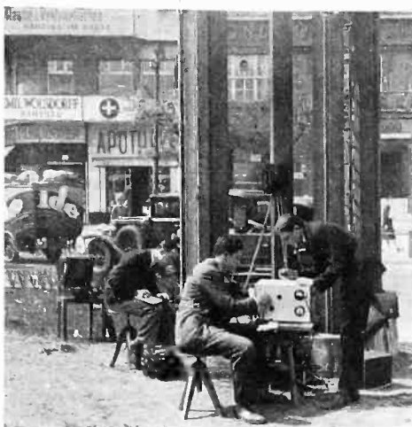
The traffic noises of Berlin being measured at the traffic-tower on Potsdamer Platz with acoustic devices
