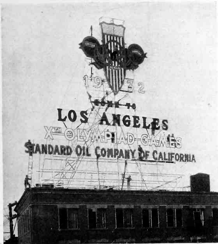
At the fall of darkness, a photocell turns on this sign. On dark overcast days it is also automatically lighted
