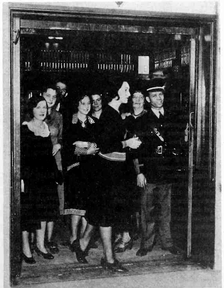
At Macy's, New York City, the elevators are safeguarded by light beams across the threshold. As long as anyone is in doorway, door can't be closed or car started. Insurance companies reduce policies 10 per cent when such electric-eye protection is provided
