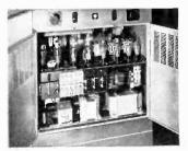
Mercury Vapor Rectifier Tubes supplying plate power for 305A Western Electric Transmitter used by New York City police.
