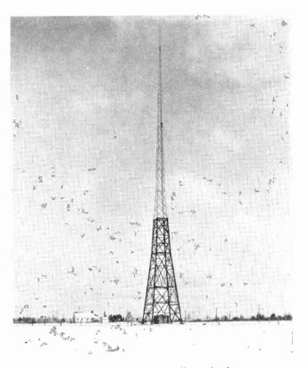
Modifying the practice of using all-wood radio towers developed in Europe (see front cover), WEBC, Duluth, Wis., has installed this combination structure, with 125-ft. wood pedestal, and total height 357 ft. A one-inch copper tube connects the tuning house with the steel radiator. Increases in signal strength have been reported.
