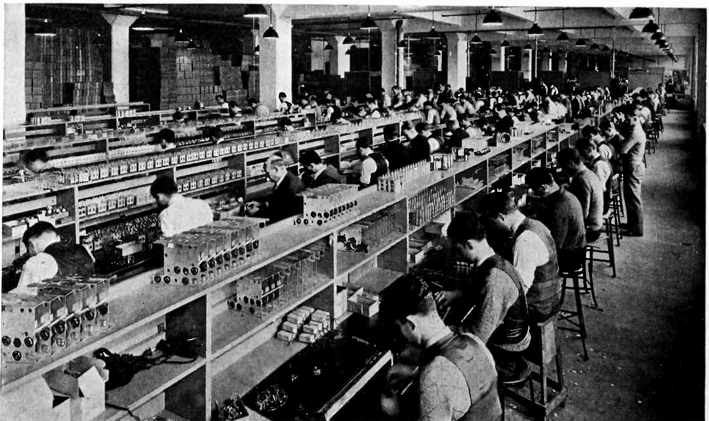
Men working at progressive chassis assembly in the Emerson plant. Here preliminary work is carried out so that sets may pass the operators at about one-minute intervals
