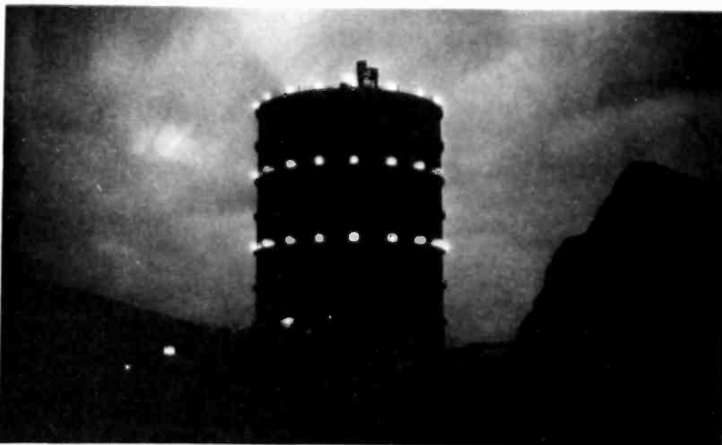
Here is a picture of the gas container of the Syracuse Lighting Company, recently described in Electronics , as photo-electrically controlled. The lamps come on automatically at dusk
