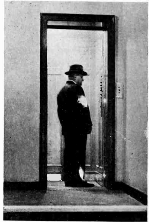
Phototubes protect occupant of push-button elevator against premature closing of doors in remodeled New York apartment
