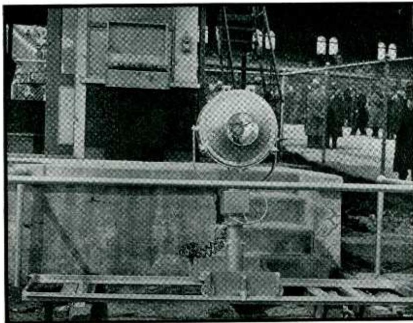
*The phototube timer, installed at the Jamaica Racetracks on Long Island, is used to trip an automatic camera at the finish of each race. The camera reveals the winner in closely contested events*
