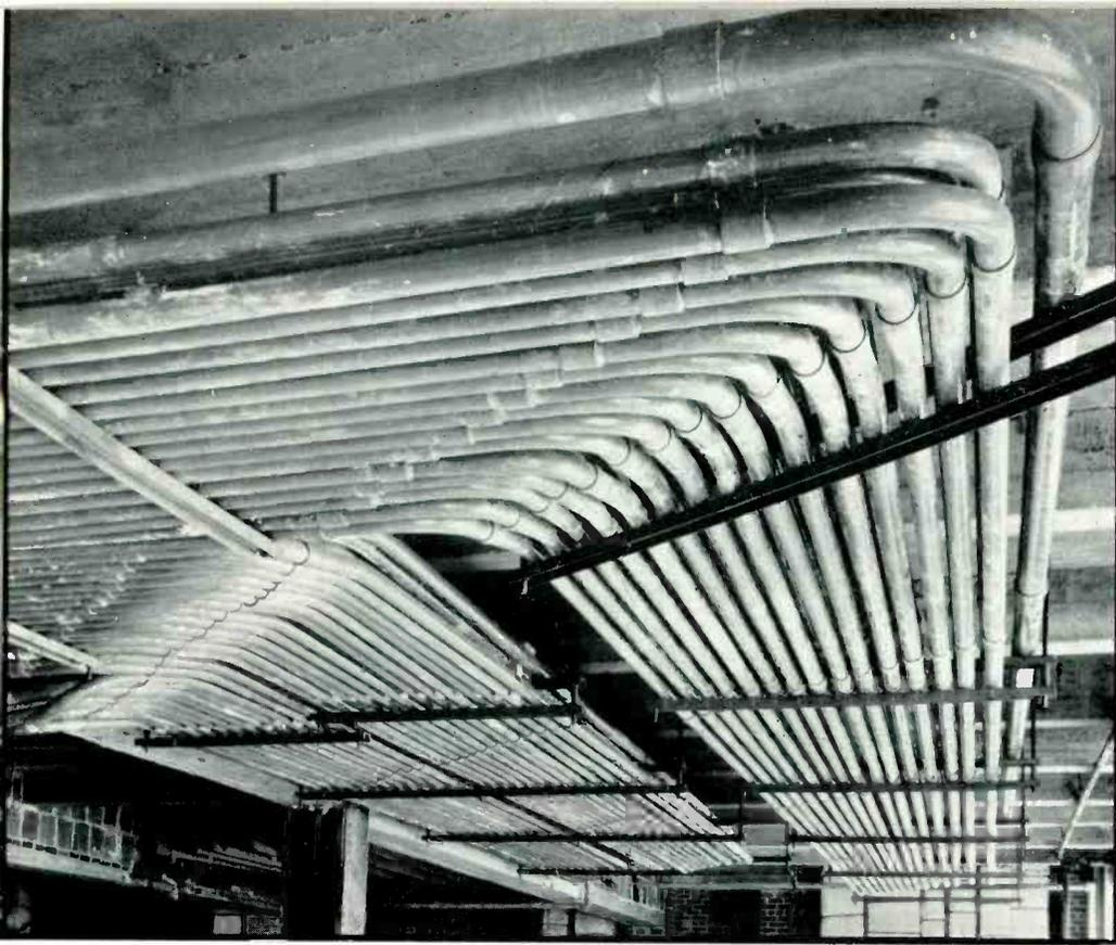
*Pipes for television: Above, 80 2-inch and 3-inch conduits installed at Radio City in 1933 for future television facilities. Below, coaxial line cords, jacks, and plugs, showing the termination of the Fifth avenue coaxial cable (main equipment room)*
