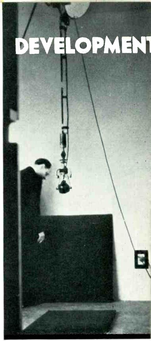
*"Pit-and-the-pendulum". Testing acoustic materials with a swinging microphone in the reverberation lab*
