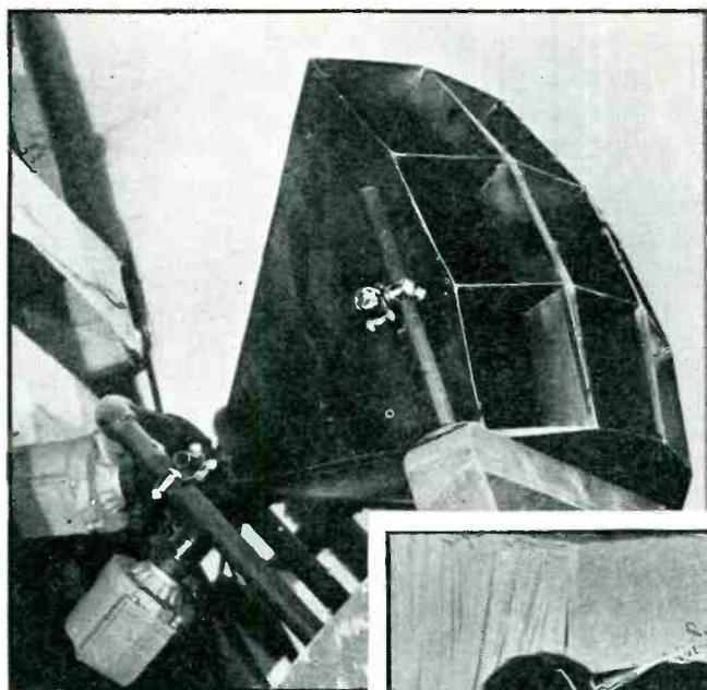
On either side of the stage are semi-circular covers extending upward 80 feet. At the base of each and facing is a group of 4 loud speakers. Sound strikes these deflecting covers, reaches the audience indirectly, providing reverberation. Below—
