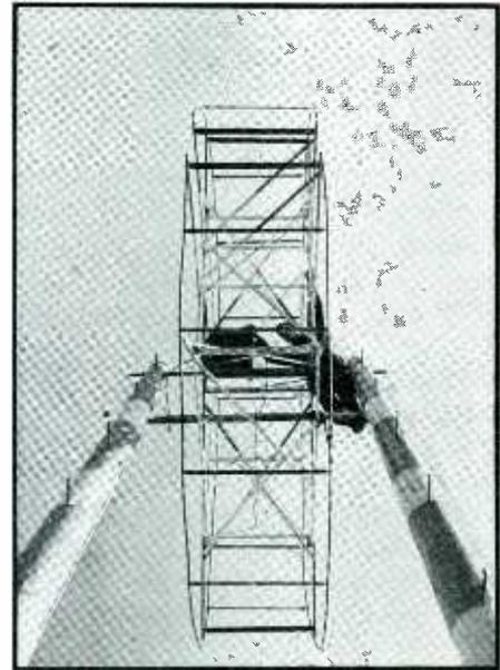
Directional "loop" antenna at the Glendale, California, airport used for sending instructions to American Airlines pilots on regular runs
