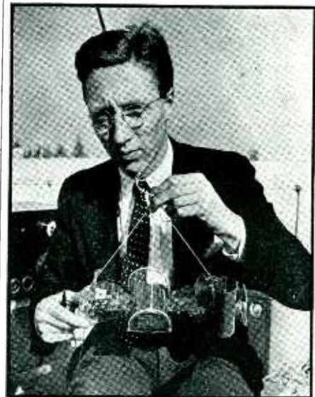
*Prof. Anthony Easton of Caltech with the one-pound radio transmitter carried aloft by a stratosphere balloon. The acorn tube delivers 1.5 meter signals, indicating wind velocity, humidity, temperature, and barometric pressure*
