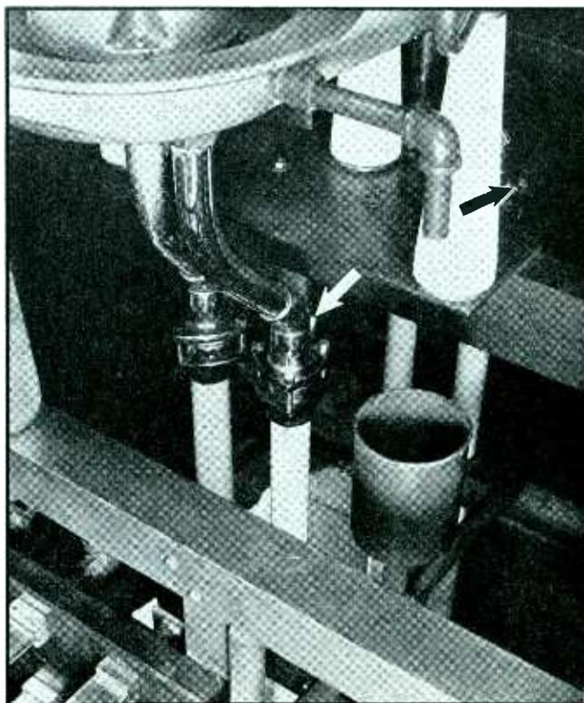
Fig. 2—Method of attaching the pipe to the water jackets. Note electrolysis target
