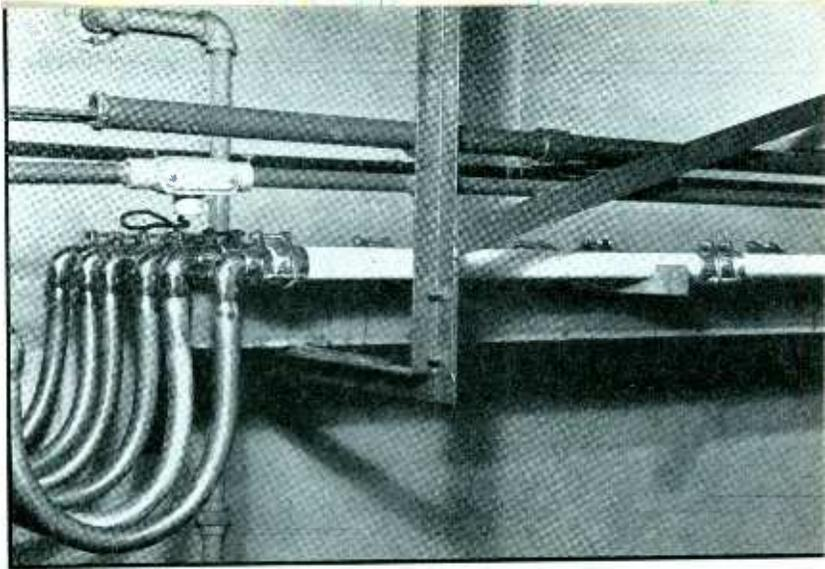
Fig. 4—Pipe ends with lead expansion loops connecting them to the pumps
