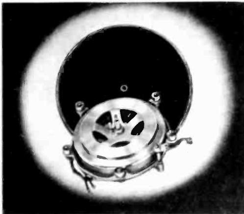
The motor is self-starting with stepless, smooth variation of speed over a wide range. One-shot lubrication through the shaft makes it unnecessary to remove the turntable when oiling. The motor is five-position rubber mounted, available in either 33  $\frac{1}{3}$  or 78 rpm, and is 4 in. high x  $9\frac{1}{2}$  in. in diameter furnished with a 12 in. Florentine bronze turntable.
