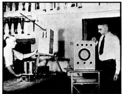
Members of the staff of the Engineering Experiment Station at Purdue are developing ultrahigh frequency directional transmitters to be used for establishing landing beams and markers for landing airplanes in fog
