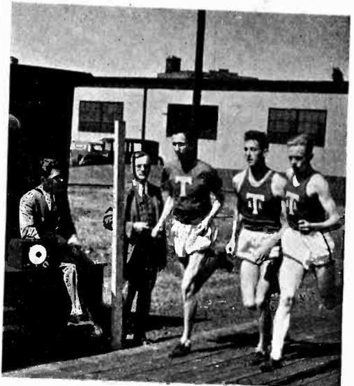
A group of track men testing out an electronic device invented by George Dadakis of the Massachusetts Institute of Technology. The track is divided into four points, at each of which a post is erected. As the runner passes the post, a bell rings. It is expected that by this method, the runner may time himself better on each lap
