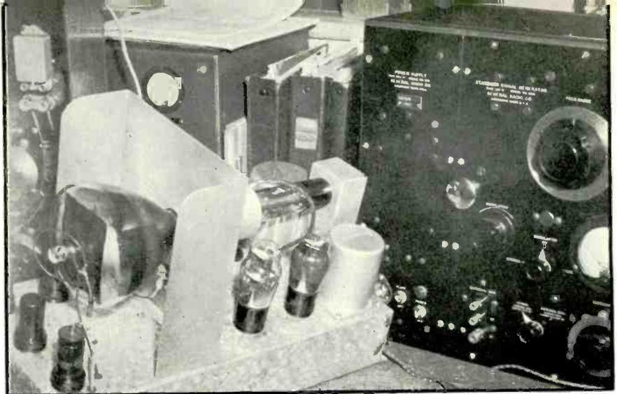
Above, the monoscope used as a source of standardized fixed-image signal for testing and alignment. A 100-watt peak video transmitter is used for testing, but not put on the air
