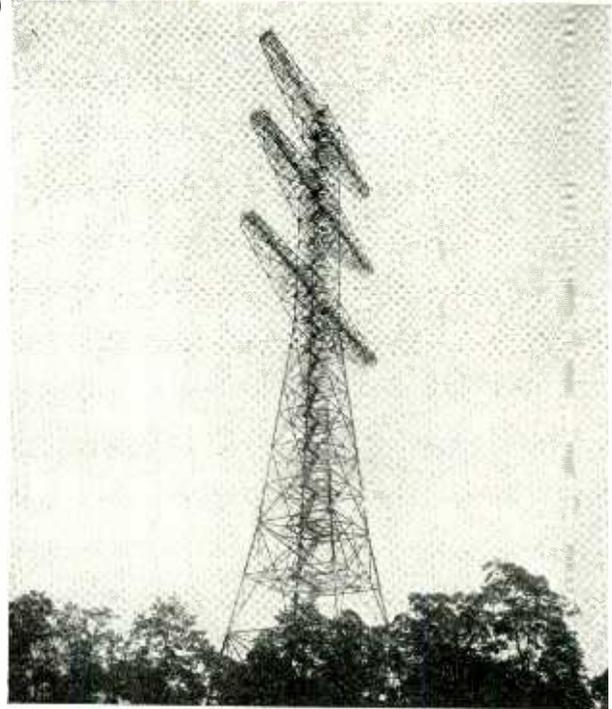
• The tower of W2XMN is 400 feet high and has "turnstile" antennae systems supported from the cross arms.
