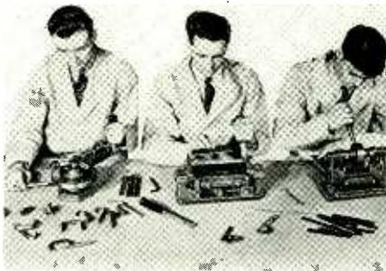
Third, the man at the left is putting a bend on each end of the channel with the bender.
