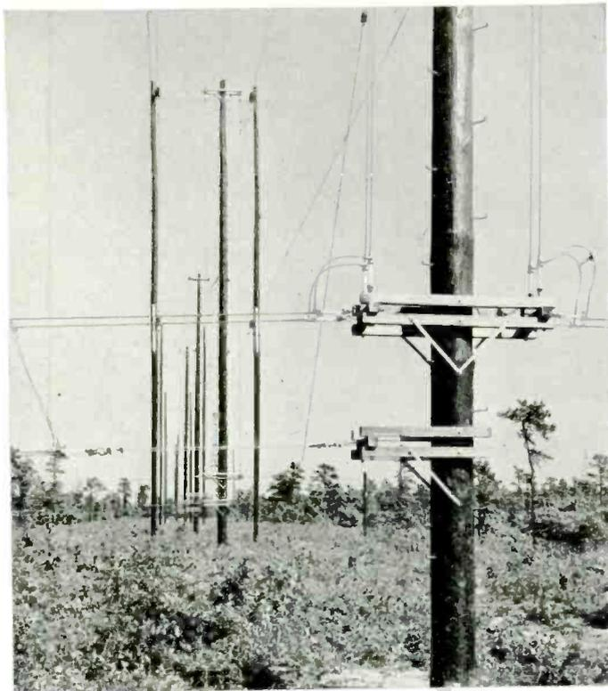
(Above) 13 DIRECTIONAL ANTENNAS are provided at the new stations, and several of them are of the four-section type shown here. Isolantite® strain insulators are extensively used in the construction of these antennas. These insulators find wide application in the radio and communications fields, because of their high mechanical strength and electrical efficiency.
