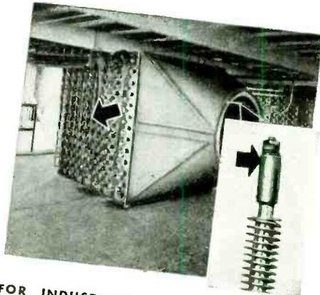
**FOR INDUSTRIAL HEATING**—Mycalex sealed terminal connectors (injection-molded) are used on many G-E Calrod heaters. The ability of G-E mycalex to withstand mechanical abuse, oil, water, and many chemical fumes make it the strongest seal available.
