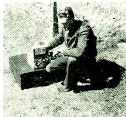
Portable 2726 kc 'phone transmitter-receiver used by Montana Power line patrolmen. It runs 2¼ watts output, weighs 22 lbs with batteries and antenna. The box on which the unit stands contains the batteries and antenna reel
