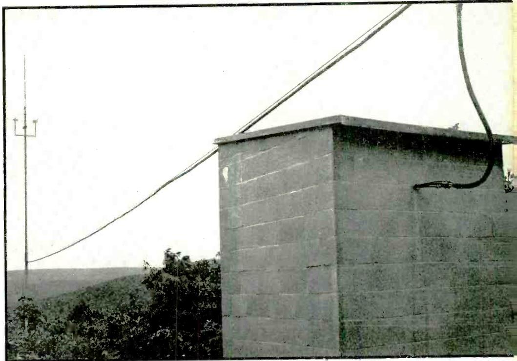
**HILLTOP REPEATER BUILDING**—One of six identical cinder-block structures. Coaxial transmission lines are bunched in a weatherproof canvas cover, divide just above the building and are carried horizontally to two antenna poles (one of which is visible here) suspended from a steel messenger cable
