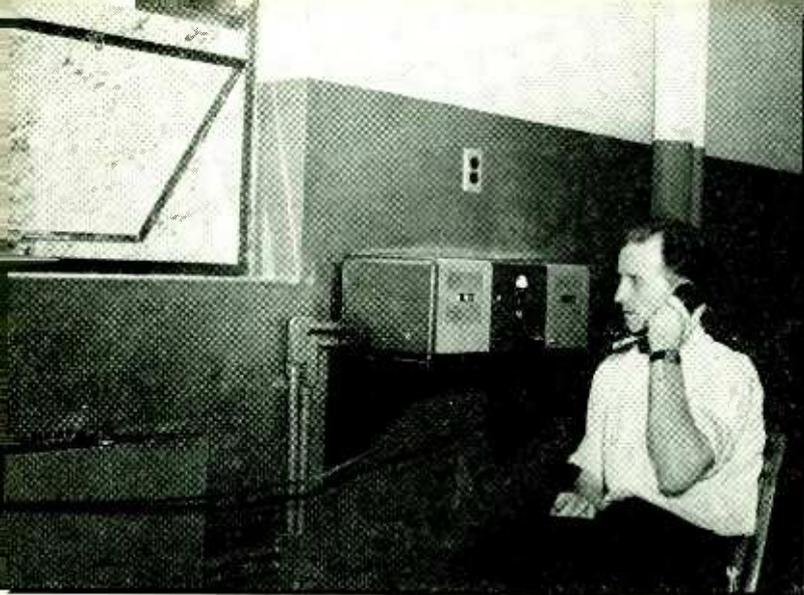
**TUNNEL PORTAL REMOTE**—This unit contains a speech amplifier and an audio amplifier and speaker. It is connected through a cable paralleling a 220-volt, a-c line (direct, or via the other tunnel portal) to the repeater station high overhead. Power and control and modulation currents go up. Output of repeater station receivers comes down. The meter is a modulation level indicator
