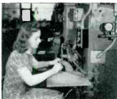
**RESISTANCE WELDING IS A HIGH-SPEED, PRECISION PROCESS** when ignitrons are used to control the high-current surges necessary for this work. There are practically no resistance-welding machines in use today that require currents higher than G-E ignitrons are able to control.
