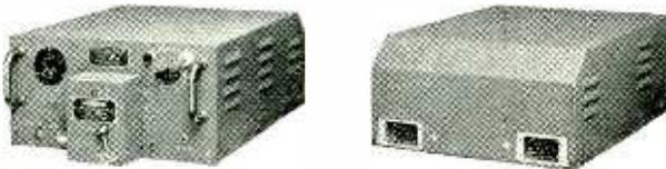
Bendix combination transmitter and receiver with two Cannon Connectors for rack use.
