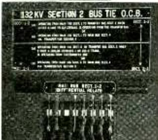
(Above) FUNCTION AND OPERATION of controls explained in detail with Engraving Lamicoid panels to minimize misunderstandings and mistakes.
