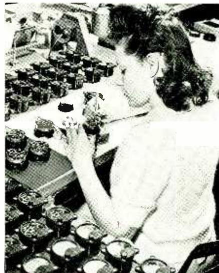
These delicate instruments which serve as the eyes of American fighting planes and bomber mechanisms pass through the hands of a Westinghouse Meter Division worker for one of the final assembly operations before the final testing after which they are shipped to the U. S. Army
