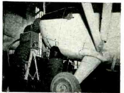
**CLEVELAND, OHIO**—Details of a gasoline heater made by Hunter and Company of this city for preheating aircraft engines quickly to starting temperatures in severe weather have recently been released for general distribution. Advantages claimed for the Hunter device are its lightness, simplicity of construction, the ease with which it can quickly be set up and taken down, and the fact that it operates on any type of gasoline at hand.
