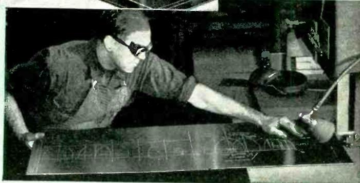
After checking the steel plate against the original drawing, it is cut to shape. The entire process, from drawing to templet is completed in only one hour.
