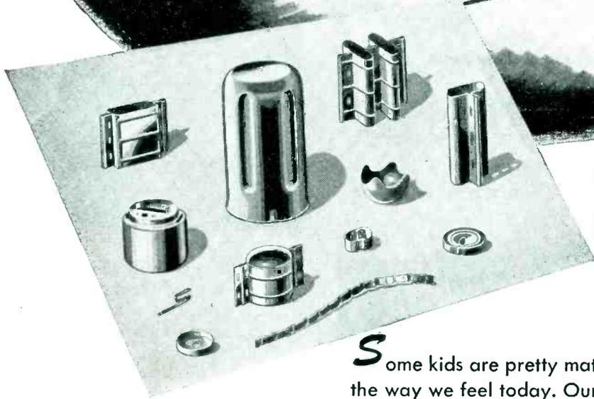
GOAT is Stamping Grounds for Small Tough Jobs. Shown are a few typical electronic tube parts that have been stamped, drawn and formed on GOAT machines, dies and presses.
