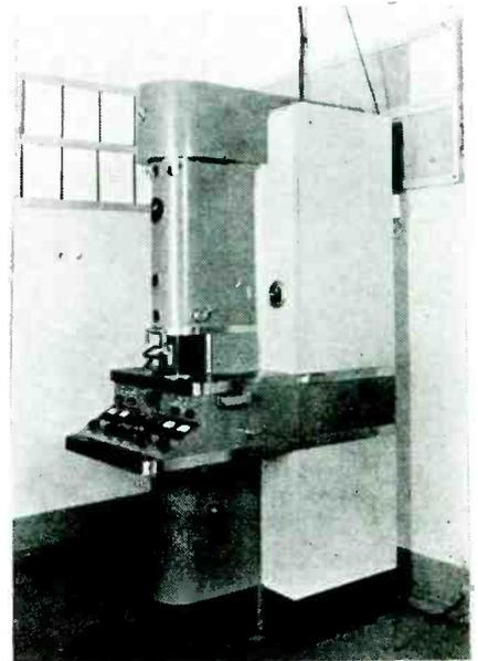
Refinements in the universal model of the electron microscope include meters at the left of the operating panel which are "coarse" and "fine" ionization gages and meters at the right which are used for maintenance checking. The image is viewed through the glass ports just above the control board. A sliding shield covers these ports for photography. This instrument contains the electron diffraction camera
