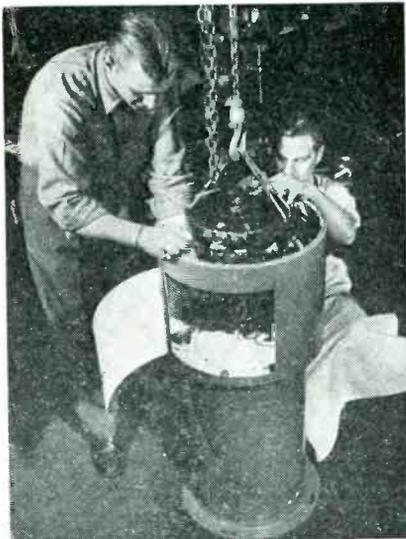
The lightweight electronic gyro-compass is fitted into its binnacle
