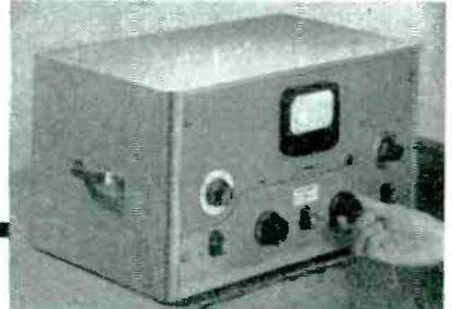
*Instruments for making over all measurements on audio equipment including total harmonic distortion, frequency response, and hum level. Model 325B Distortion Analyser illustrated.*
