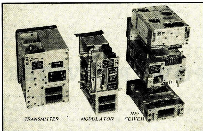
This FuG 16Z German aircraft radio command set is divided into five individual magnesium alloy castings fitted together by means of dowel pins and electrical plugs and jacks
