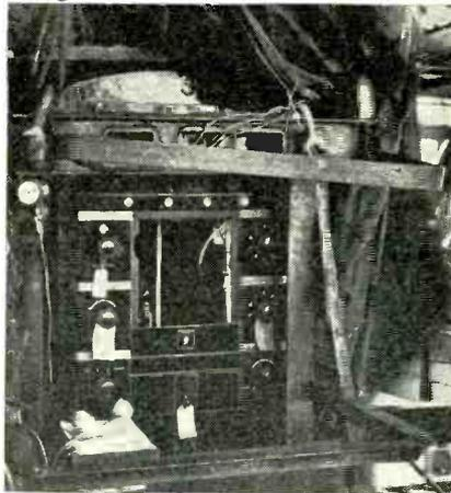
View of the x-ray control panel hanging at one of the skyscraper levels. Colored signal lights replaced the doubly insulated telephone for communication with operators at the tube head when construction noises were too great
