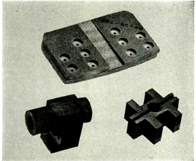
Panelyte, the structural laminated plastic, is both versatile and adaptable. Close tolerance work is possible because sheets are thoroughly bonded and the structure homogeneous. Irregularity of shape or intricacy of design are not obstacles, as parts are lathe turned, milled or drilled to exact specifications.
