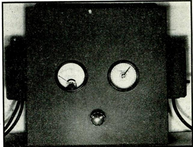
Complete electronic thermometer. The dial at the right is mechanically coupled to the potentiometer used for establishing the control point, and the meter at the left indicates temperature deviation in degrees above and below control point
