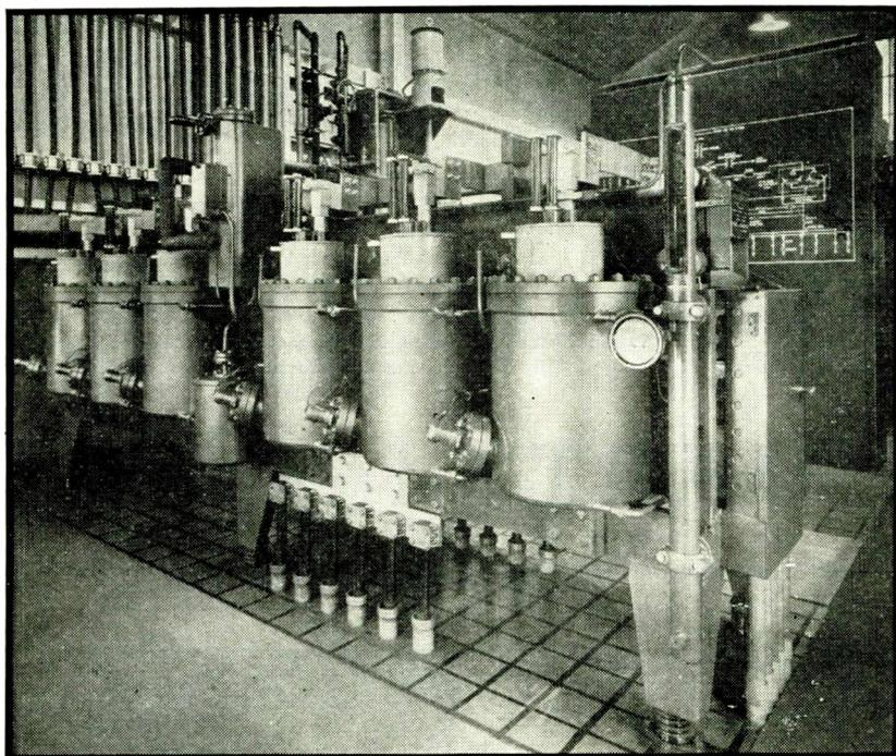
Ignitron mercury-arc rectifier equipped with an industrial type vacuum gage having a handwheel and pinion for operating the mercury plunger. The gage is at the extreme right
