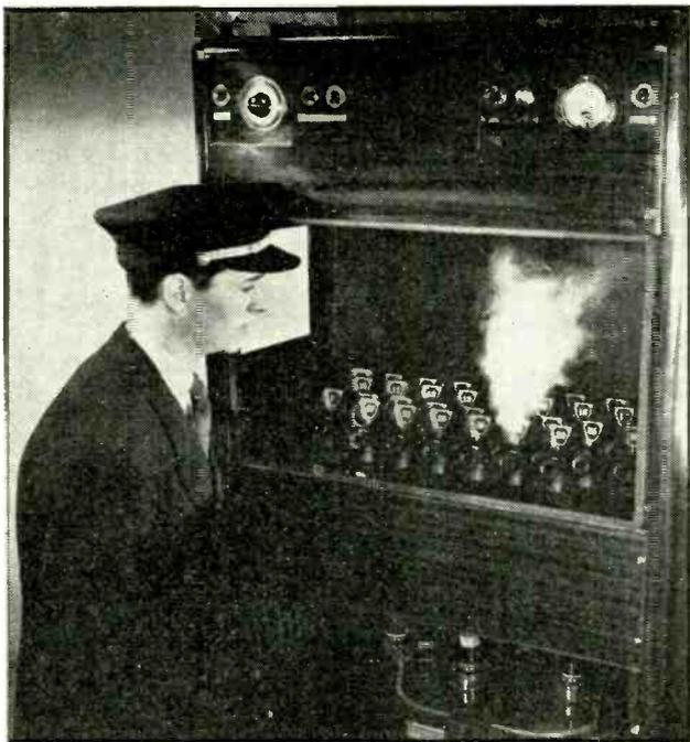
Numbered pipe outlets in the smoke-detecting cabinet show the ship's officer at a glance which space is afire when the photoelectric cell sets off the automatic alarm in the Rich-Audio fire-detecting system made for ship use by Walter Kidde & Co., Inc., of New York
