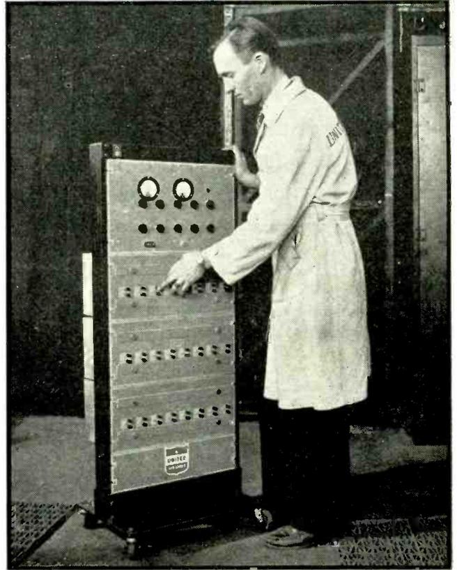
Signal generator used for measuring frequencies and aligning all aircraft radio receivers carried aboard Mainliners. Push-buttons select any of 24 crystal-controlled frequencies
