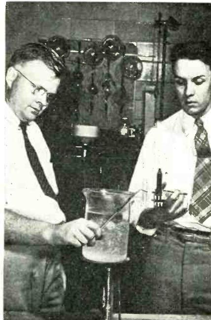
Dr. Reid Fordyce and Dr. David T. Mowry, co-discoverers of Cerex, hold up for comparison two radio parts. Although identical in size and shape before immersion in the boiling water, the ordinary plastic (left) wilted and shrunk, while the black Cerex part was unaffected by boiling water
