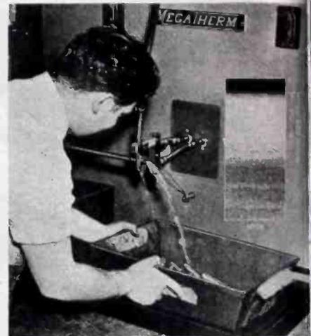
Case-hardening of chromium-molybdenum steel bearing pins with a 5-Mc r-f generator. Inset at right is a micro-photo of the hardened surface. The white portion is the outside case which has a thickness of 0.025 in.
