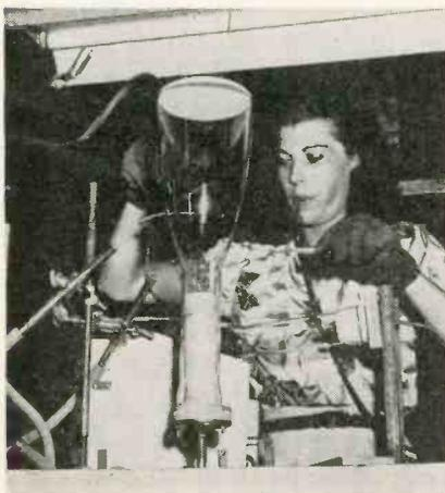
Metallic buttons are sealed-in on cathode-ray tubes at the Dobbs Ferry plant of North American Philips. The operator controls the air pressure in the tube with her mouth while the gas burner is rotated around the button
