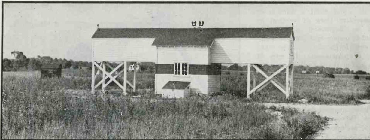
Building housing runway localizer antennas and associated transmitter equipment
