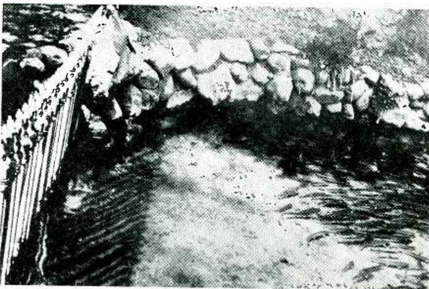
Fig. 1—Young rainbow trout in an irrigation canal swim away when they come within the zone of influence of the electric fish fence at left. The rod-type fence is controlled by a special electronic generator and emits electrical charges that repel the fish without harm
