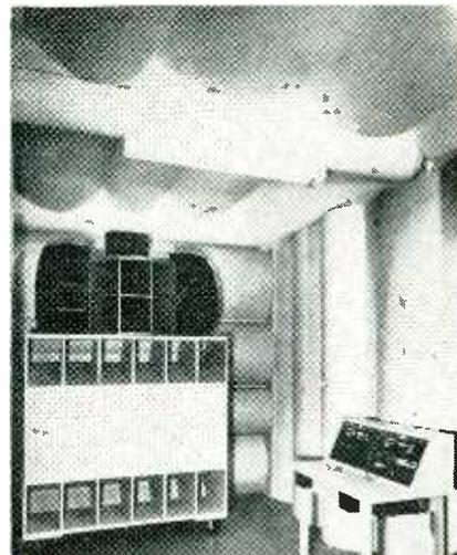
Diffuse sound room in the Electro-Acoustic Laboratory of Harvard, where noises heard in a plane during flight are realistically reproduced
