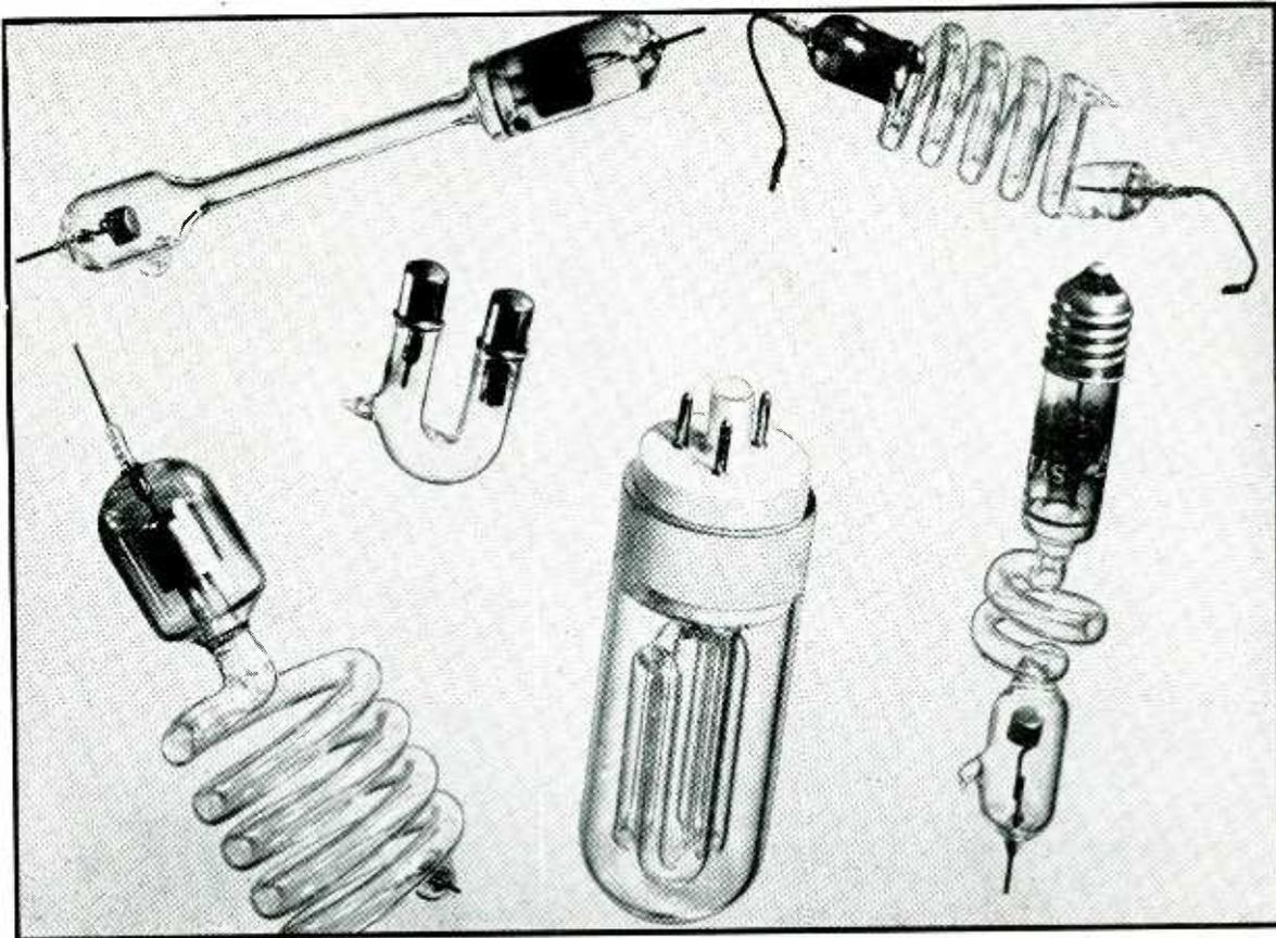
Examples of externally-excited gaseous discharge tubes
