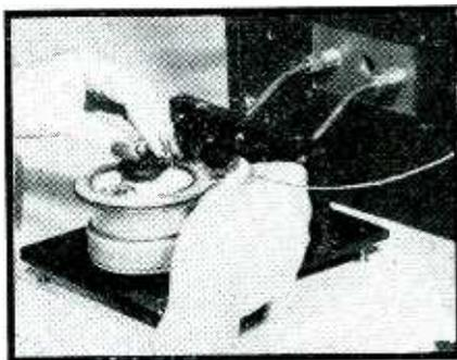
R-f soldering of metallized edge of glass window to case of meter, using a single-turn flattened work coil
