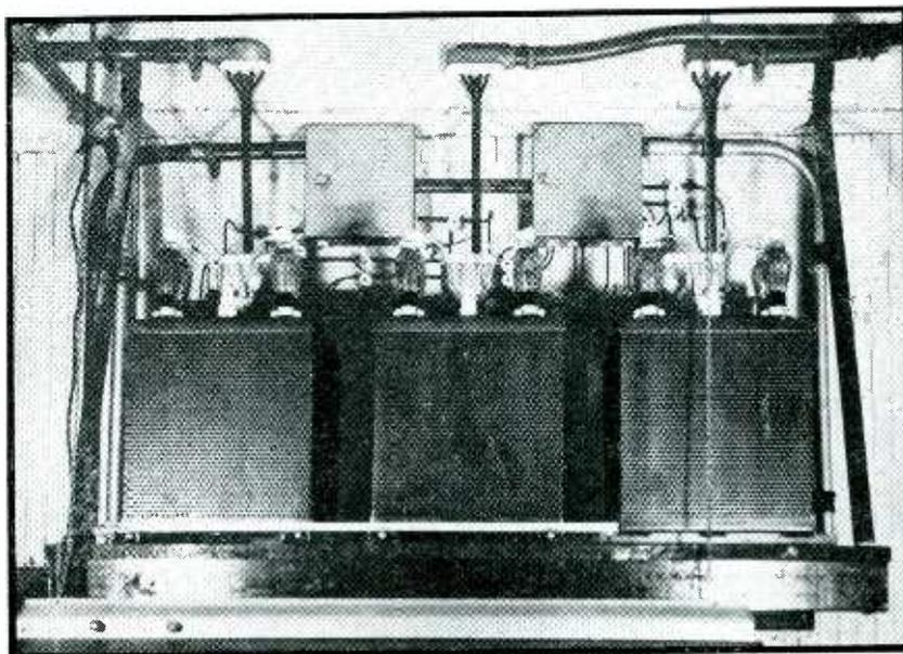
Master power supply, using twelve type 866 mercury-vapor rectifier tubes to supply 1,500 volts d-c to as many as ten r-f generators scattered throughout the plant
