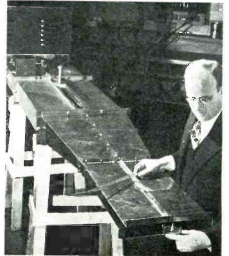
Use of a waveguide as an electronic blow torch to project high-frequency energy into materials is demonstrated at the Westinghouse Research Laboratory by Dr. J. A. Hutcheson, associate director. Liquid plastic in the dish can be solidified in three minutes
