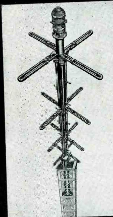
**1—VERY BROAD BAND** — incorporates features of ordinary turnstile with vast improvement of FOLDED DIPOLE principle.
