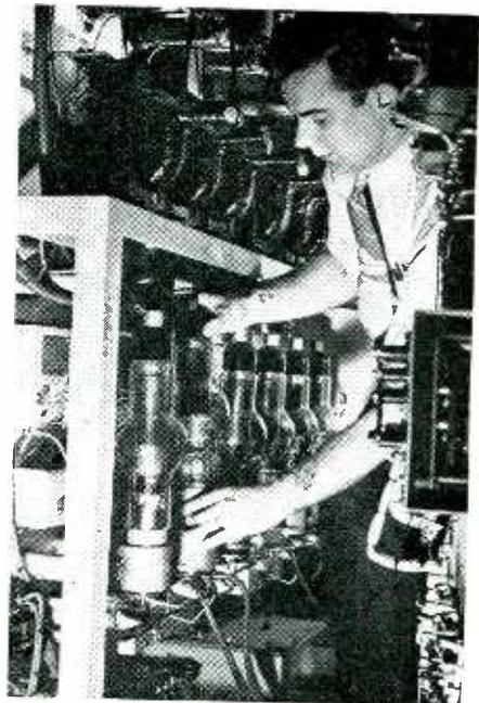
An engineer checks one of the rectifier tubes in the electronizer vulcanizer developed by Westinghouse for the Firestone Fall River, Mass. plant
