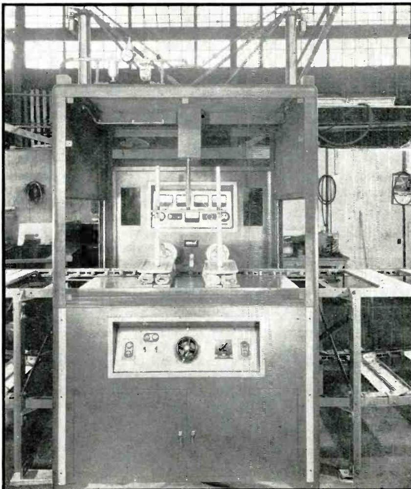
FIG. 2—Adaptation of the equipment, used here for preheating tank treads, to different types of work is possible by modifying the heating electrodes. The work and indicating meters are visible to the operator through a protecting screen not shown here
