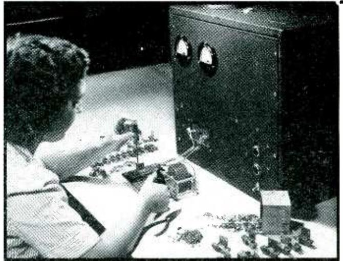
R-f soldering of pole faces to Alnico magnets of meter movements
