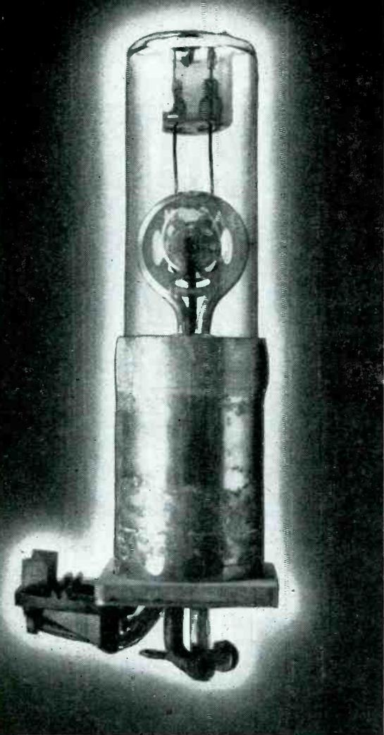
Type M-312 water-cooled 10-cm transmitting magnetron employed in Japanese naval search radar
