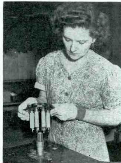
Eight elements for test equipment gear are assembled with a preformed ring of solder in position at the juncture to be sealed, then secured in a fixture. The operator lowers them through the holes into the field of an induction coil connected to a 15-kw RCA r-f generator used in the Camden plant of RCA Victor Division
