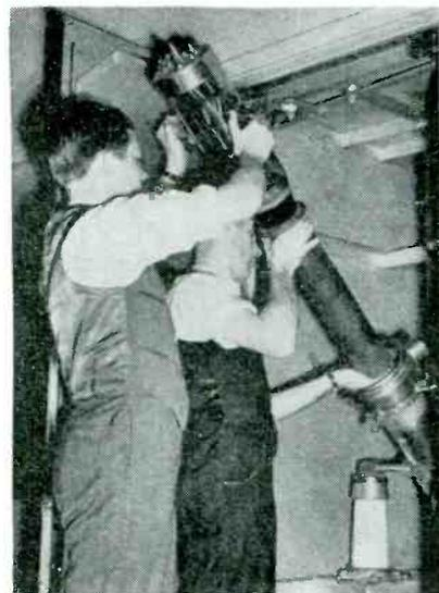
Two engineers install one of the 100-kw water-cooled transmitting tubes at the Government-owned short-wave station in Canada. A special beam antenna gives a total effective power of 10 million watts to the station
