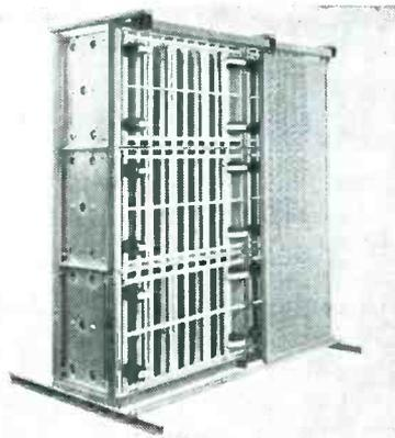
(illustrated). Although the equipment is used most advantageously when placed in the incoming air duct supplying a space, room-type units are also being manufactured which by recirculation withdraw most of the impurities from the air.
