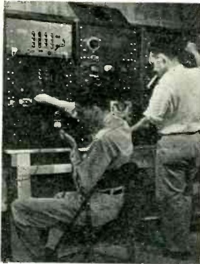
Master control room for V-2 tests, in blockhouse with concrete walls 10 feet thick. Each rocket has 20 channels for sending back by radio and radar the readings of the various instruments being carried into hitherto unexplored regions of interstellar space
