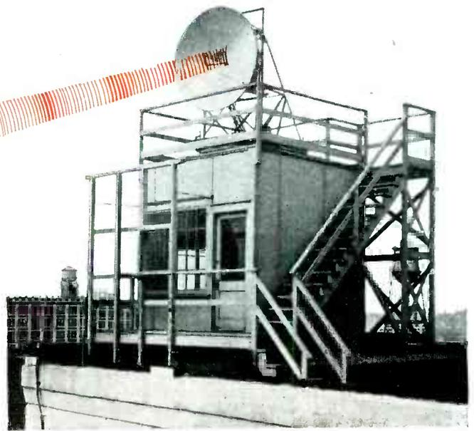
A radio link between remote pickup and studio or between studio and transmitter
