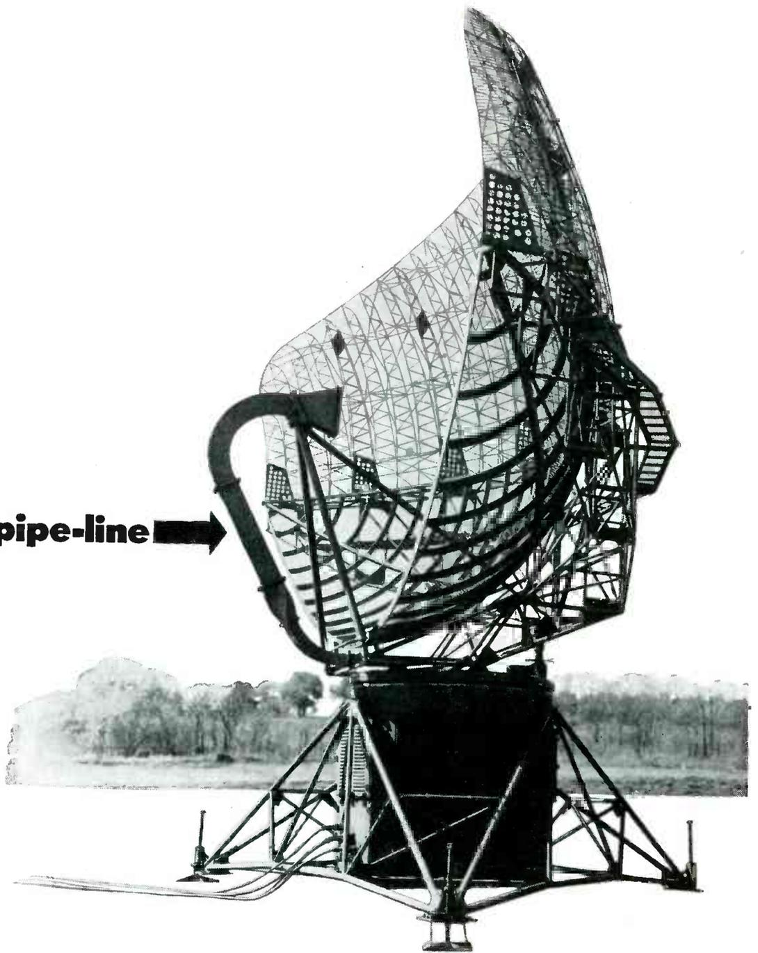
Microwaves make their journey from apparatus to antenna not by wire, cable, or coaxial — but by *waveguide*.
