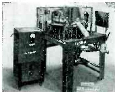
24 Head Radio Tube Exhausting Machine.
