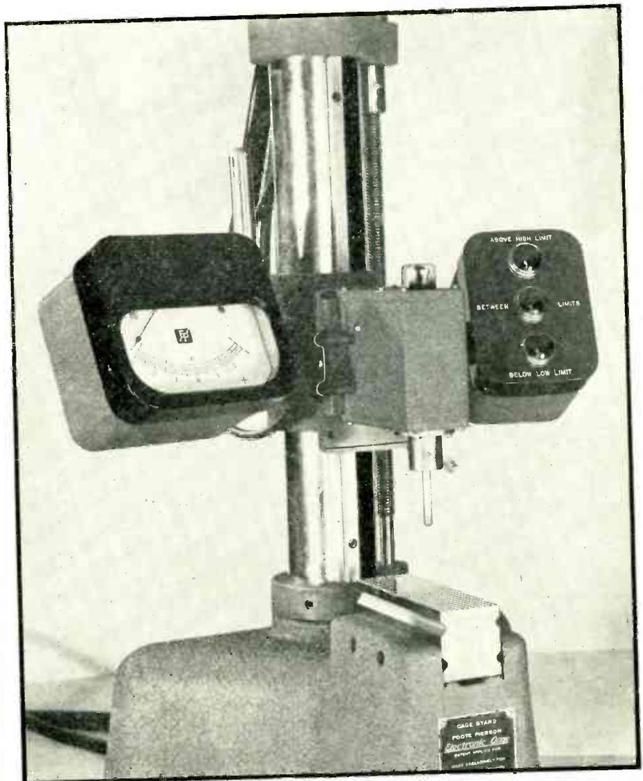
The gage stand, showing the diamond-point contact, indicating meter, and limit lamps
