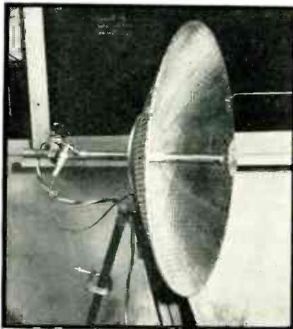
Rotary wave radar unit using two-foot diameter reflecting dish arranged as in Fig. 2
