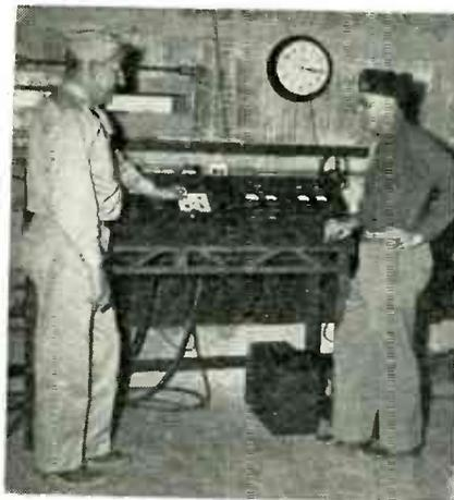
Control desk from which rocket can be fired and its fuel cut off by radio if trouble develops during flight
