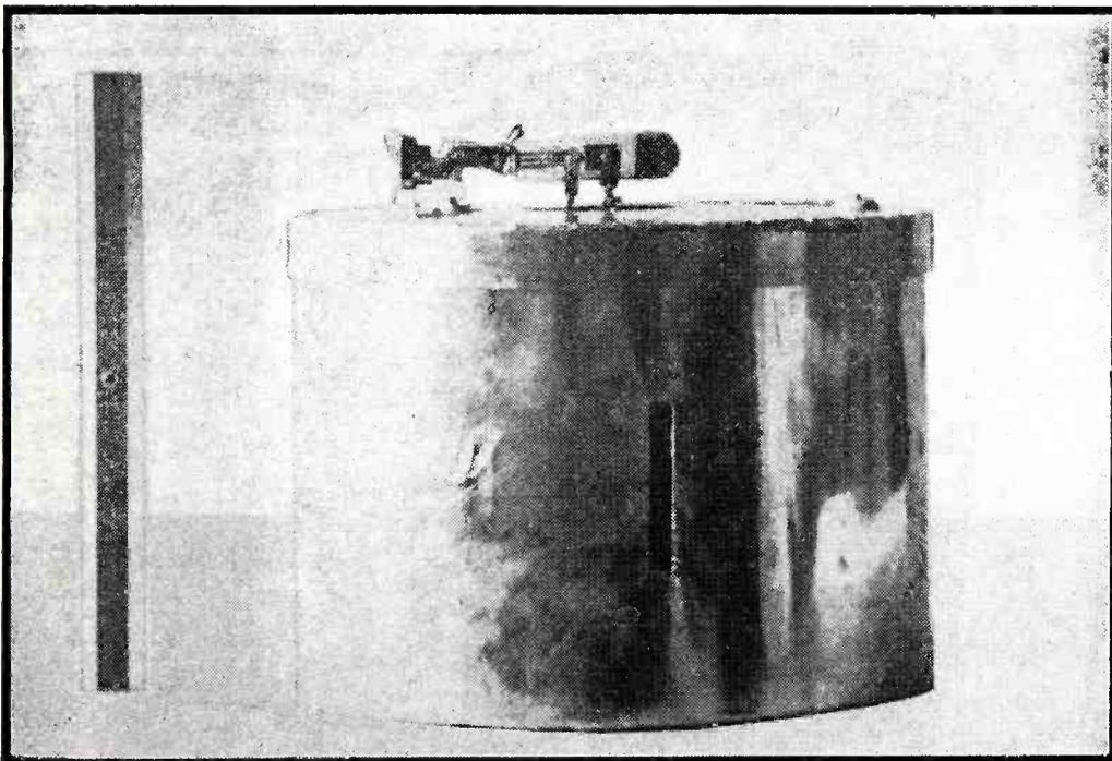
Uhf oscillations are obtained from negative-grid triode by inserting the transmission line tank into a cavity resonator
