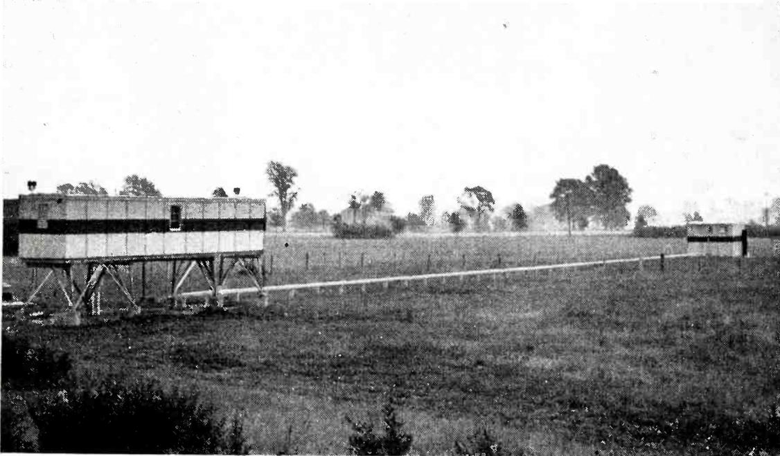
CAA instrument landing installation at Indianapolis. Antenna building is at left, in line with the end of the runway, while transmitters are in smaller building at right and 300 feet away
