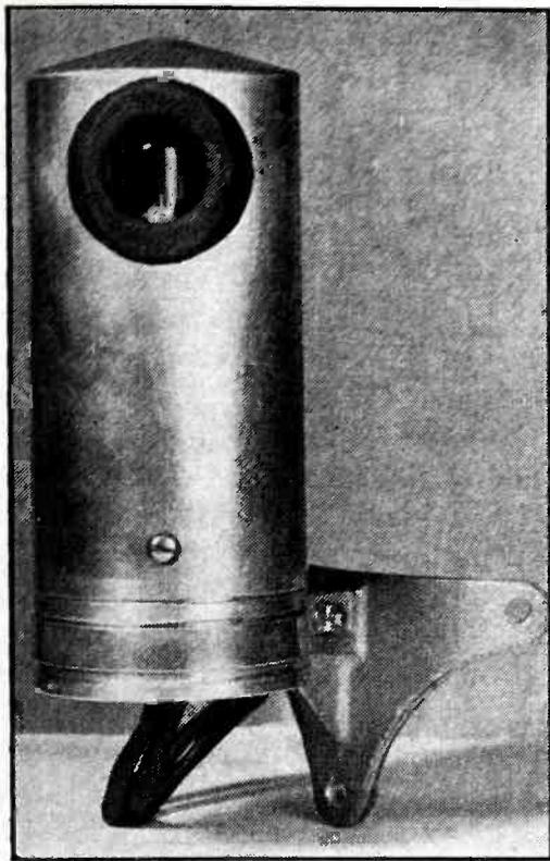
Sunswitch suitable for mounting on a street lighting system pole
