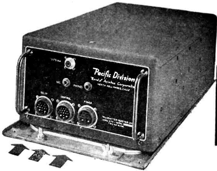
Photo courtesy Pacific Division Bendix Aviation Corp., North Hollywood, Calif. Transmitter-Receiver Unit for mobile communication equipment. Model LTR-1
