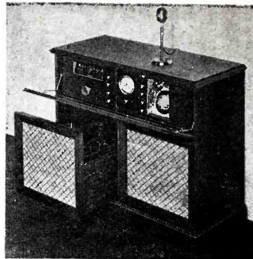
switch and broadcast receiver, making possible the automatic recording of programs in the absence of the set owner. In addition, a disc record album can be continuously embossed on the film from the turntable and pickup with which the console is equipped. Other recorders suitable for office and home use are also available.
