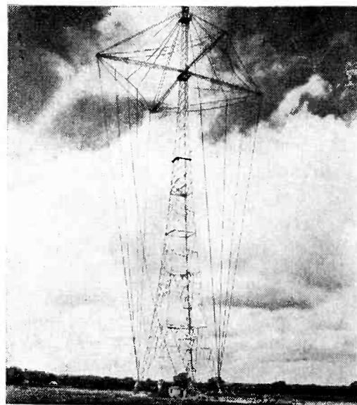
Antenna system and transmitter building of the Red slave station of the new Decca system at East Hoathley, England
