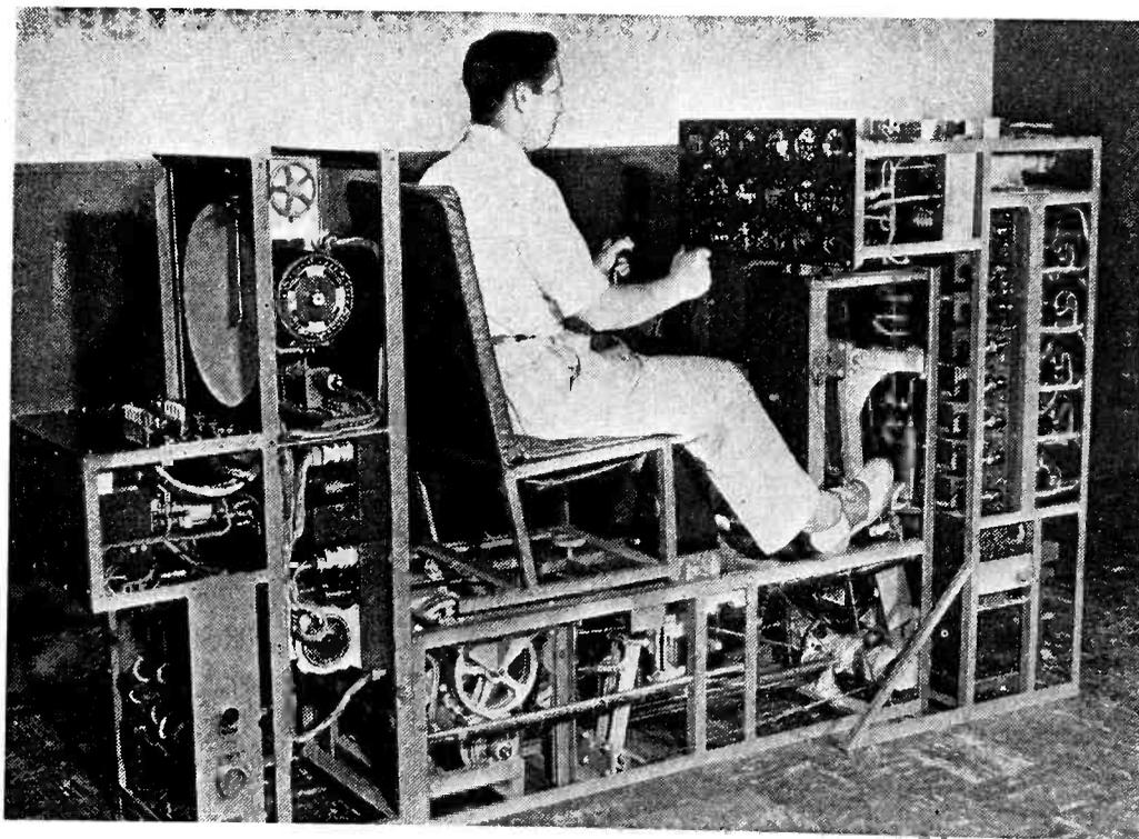
Flight characteristics of an AT-6 airplane in the air are simulated by the prototype version shown above stripped of its aluminum fuselage. Produced for the Army Air Forces by Curtiss-Wright, it uses servos to feed an electronic computer
