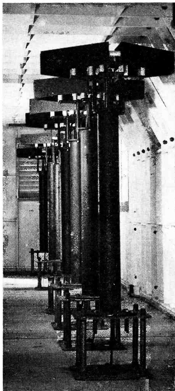
Inside of antenna building, showing array required to produce a straight localizer course. Technical details of this system were given in the February and March 1945 issues of *ELECTRONICS*
