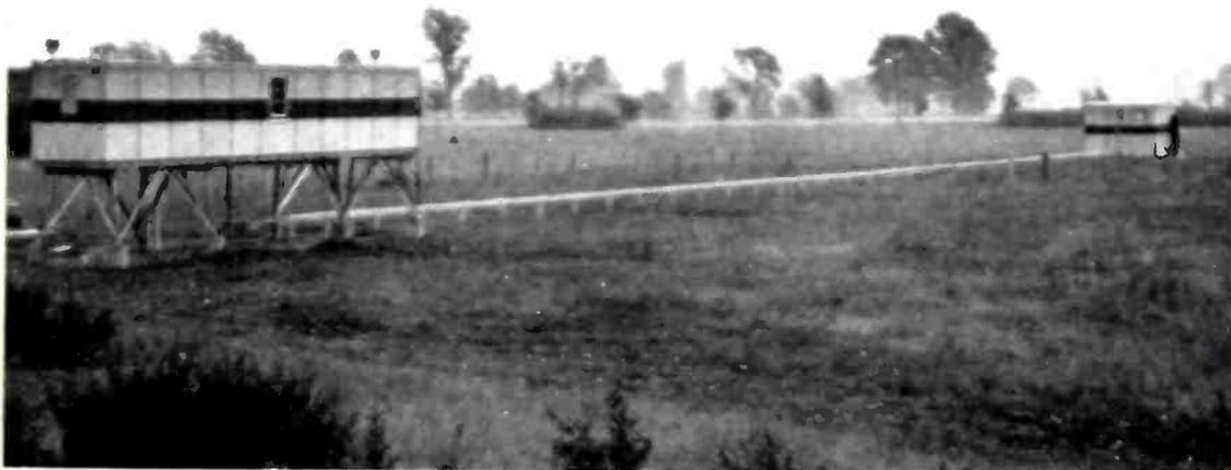
CAA instrument landing installation at Indianapolis. Antenna building is at left, in line with the end of the runway, while transmitters are in smaller building at right and 300 feet away
