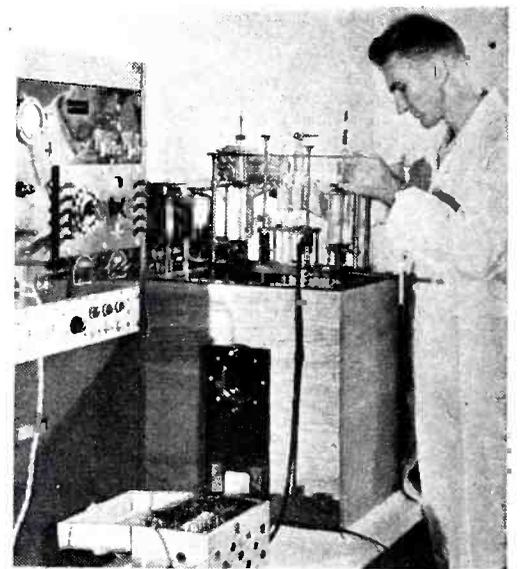
Fig. 2—Research technique is done on a production basis using an electronically regulated voltage source to maintain the same accuracy as under laboratory conditions
